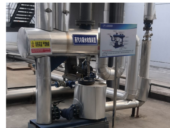
Steam condensate recovery system
