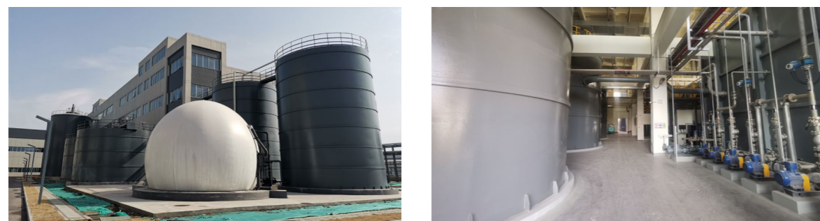
Upgraded sewage treatment stations
